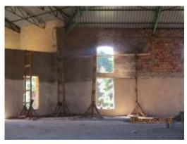
After furlough, one of our first projects at Galilee UMC was to connect the highest section of the walls to the roof structure, a job of two and a half weeks. Once the walls were secured, we purchased almost all of the available cement in Kasenga and began plastering the walls. The walls are expansive, so the work took almost a month!
